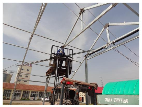
Fix D2 by No.D34, D30, D32. Fix No.D1 3" side track & vertical track to upright. Connect No.D2 and No.D1 by No.D33
